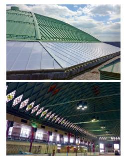
The Playland Ice Casino's new metal roof with the Horizon C-Series translucent polycarbonate canopy system lighting the diamond windows along the perimeter.
