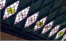
The old rubberized fabric perimeter was not energy efficient and provided very little natural daylight compared to the new Horizon C-Series system.
