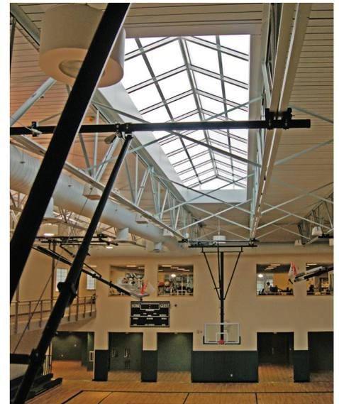
The original fiberglass panels were yellowing, delaminating, and preventing much sunlight from entering. The new S-Series polycarbonate skylights let in so much light, electric lights can be turned off on sunny days.
