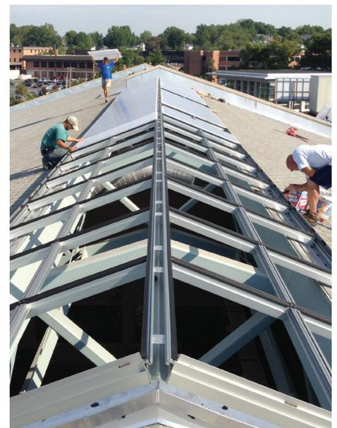
The S-Series structural ridge skylight, constructed with the Pinnacle 350 framing system, offers durability, large span capability, and fast on-site assembly.
