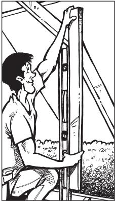
Locate the two bottom corners of the skylight opening on the underside of the roof deck, relative to the ceiling opening and type of well. Mark these points on the roof by driving nails through the roof deck. Measure up from the two nails the appropriate distance as required by your unit (refer to Sketch 3) to locate the top corners of the roof opening and mark them with nails also.
