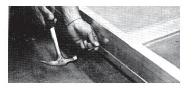
**STEP-8:** Apply silicone sealant at interior of all perimeter sill splice locations.
