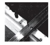
**STEP-5:** Install rafter bars over rafter channels. Ensure that centerline of rafter bar aligns with scribe on line on sill. (see illustration below). Install purlin bars over purlin channels. Ensure that centerline of purlin aligns with scribe line on rafter bar. (see illustration below). Fasten rafter and purlin bars with #14 x 1 self-drill/self-tap screws thru predrilled holes in rafter and purlin bars.
