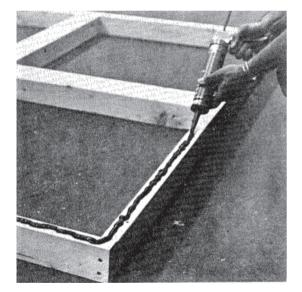
**STEP-1:** Before installation of unit, ensure that the building curb has been properly prepared to receive unit. Place a bead of sealant on top of flashed building curb (see illustration at left, flashing omitted for clarity).
