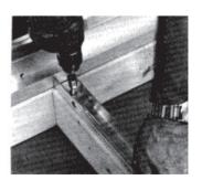
**STEP-4:** Install aluminum channels for purlin bars. Ensure that centerline of channel aligns with centerline of support and that ends of channels are 1/2" away from face of rafter channels. Secure Aluminum channels with 1/4" dia. X 1 1/2" stainless steel lag bolts (not provided by Wasco).
