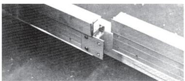
**STEP-3:** Install aluminum channels for rafter bars. Ensure that centerline of channel aligns with centerline of support and scribe mark on sill. Secure aluminum channels with 1/4" dia. X 1 1/2" stainless steel lag bolts (not provided by Wasco).
