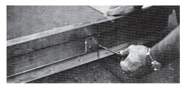
**STEP-7:** Anchor perimeter sill to building curb with 8d stainless steel or galvanized nails (not by WASCO).
