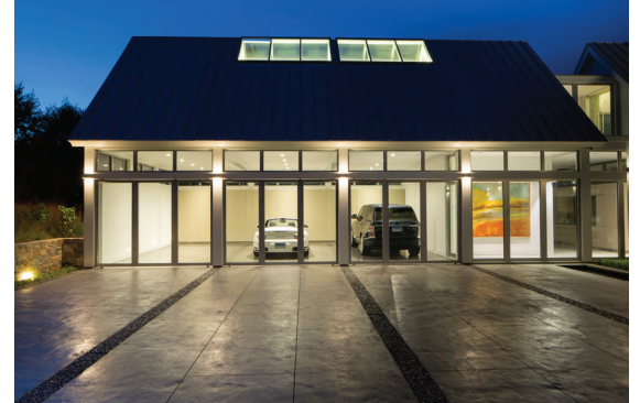
There are no steps. The house sits on thermalized plinth stone inside and out so it's warm underfoot inside and melts the snow outside.
