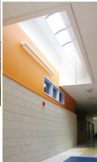
Natural light comes into the main lobby and hallways from the Double Dome Barrel Vault skylights above.
